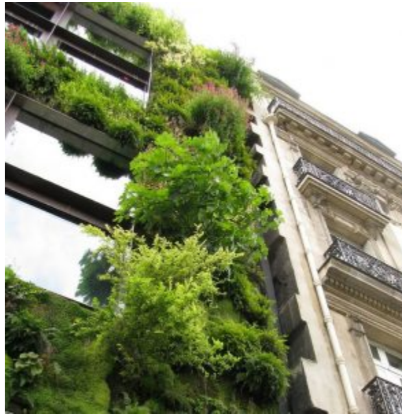
Figure 9.2 Example of a living green wall
