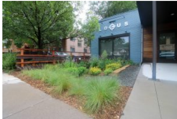
Figure 9.4 Example of a rain garden
