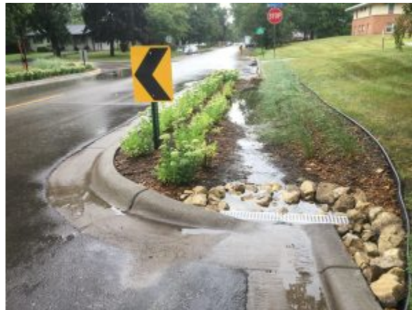
Figure 9.3 Example of a vegetated bioswale
