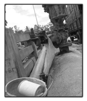
Figure 6.1 Leaky water pipe in south Bengaluru (Bangalore). Source: Sadoway, Gopakumar, and Sridharan (2013).
